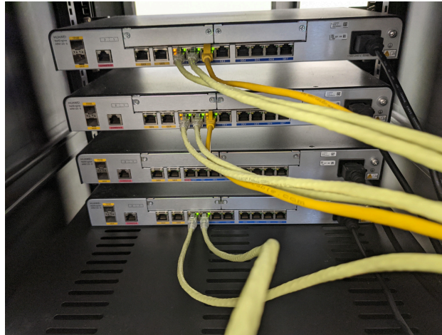
Figure 6: 机柜背面接线图
